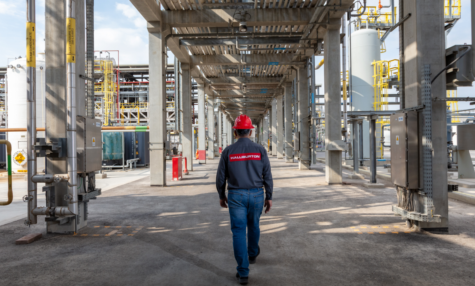
Halliburton chemical reaction plant in Saudi Arabia
