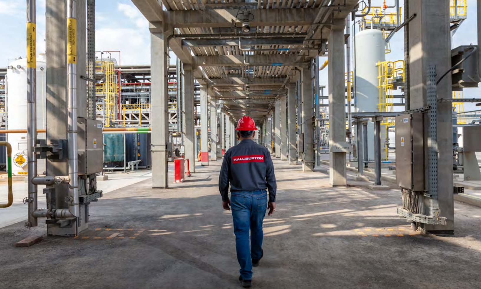
Halliburton chemical reaction plant in Saudi Arabia
