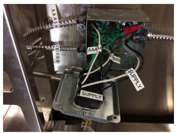
MAIN ELECTRICAL BOX SHOWING SUPPLY LINE ENTERING ON RIGHT SIDE OF BOX.
