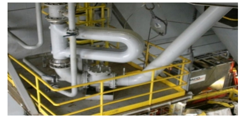
A Coriolis flow meter and flow diversion.
