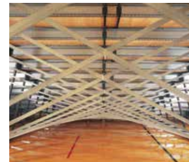
G. Tension Bracing Through bolted to the frame to provide additional stability. All bracing is coined to remove sharp edges, and all ends are rounded for safety.
