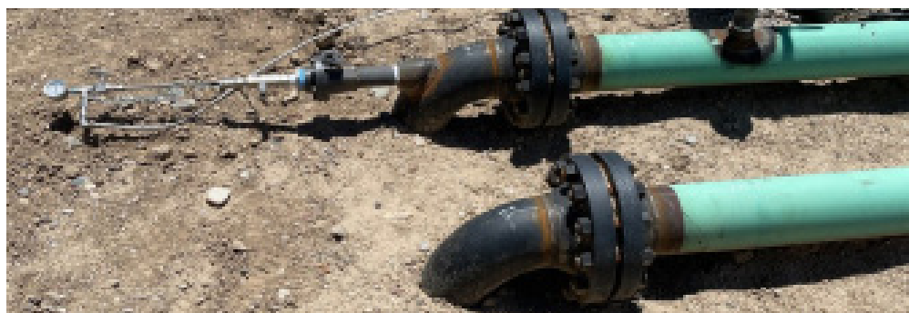
The atomized injection point for H 2 S Scavenger on the new retention loop.
