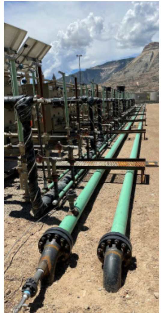
The loop was built above ground to limit construction costs and make it easier to inject chemicals and monitor gas flow.
