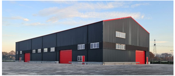
The opening of a new service center in Emmen, Netherlands, demonstrates our unwavering global commitment to geothermal energy initiatives.
