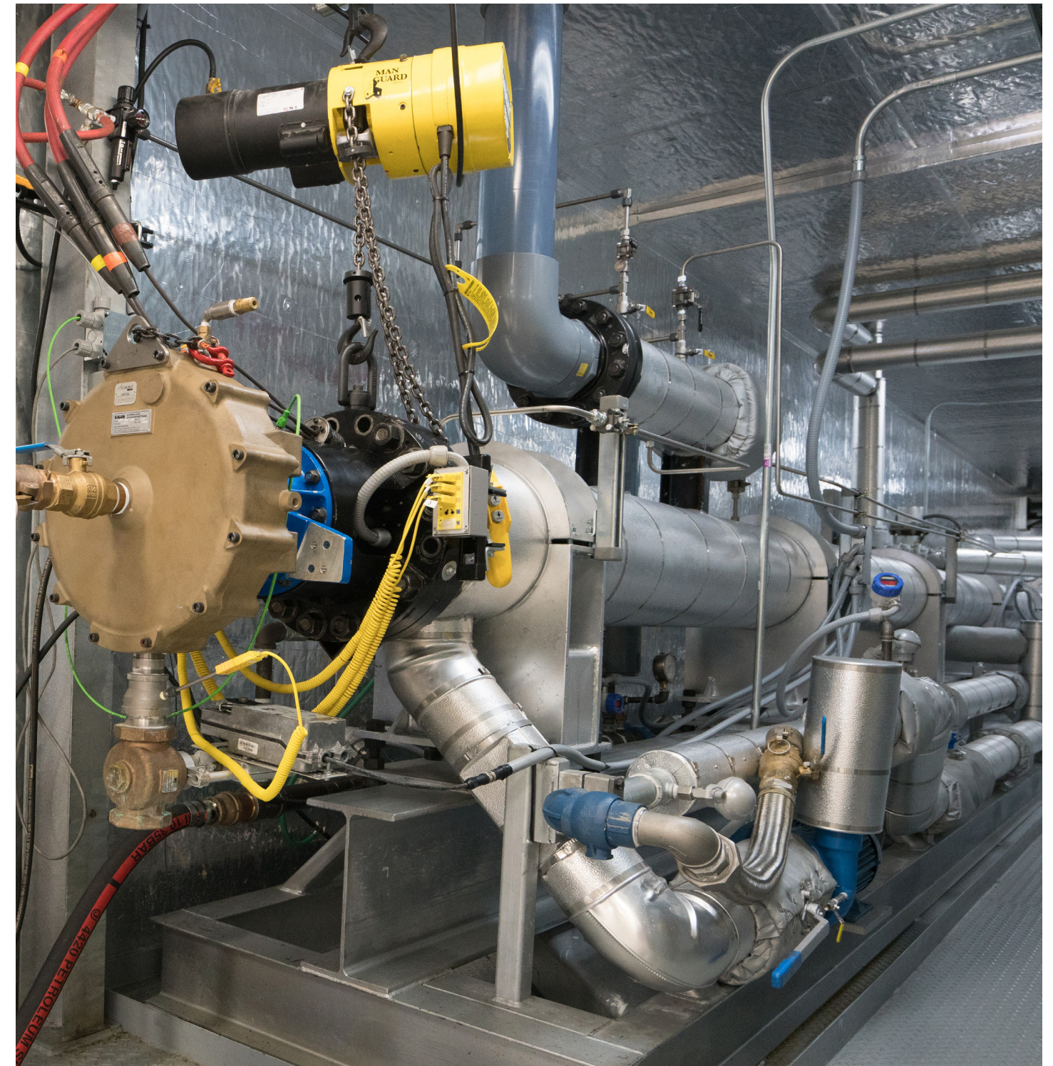
Motor dynamometer test loop: Used for qualification and validation of all motor design implementation.
