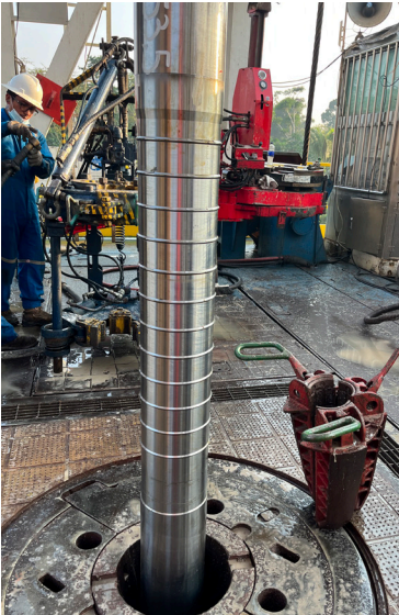
Liner hanger prior to run-in-hole
