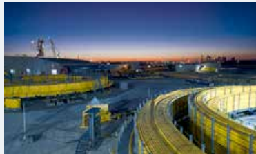
Aker Solutions’ umbilical facility in Mobile, Alabama, with its high-capacity horizontal cable, is specially designed to meet the challenges of demanding deepwater applications.
