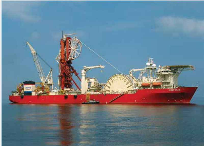
The Deep Blue is one of the most advanced pipelay and construction vessels of the subsea industry and the flagship of the Technip fleet.
