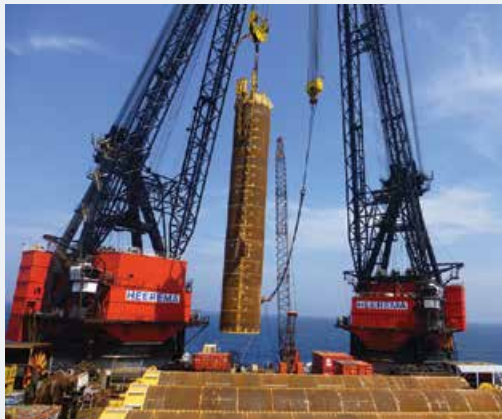
DCV Balder lifting a Jack/St. Malo suction pile.
