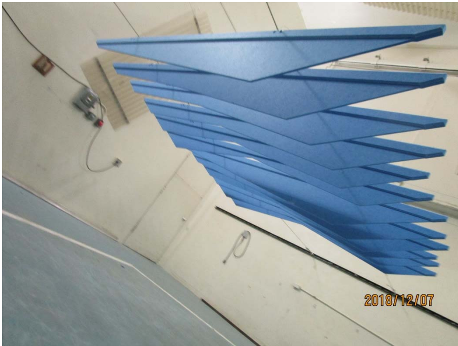
Figure 2 - Detail of varying baffle depth profile
