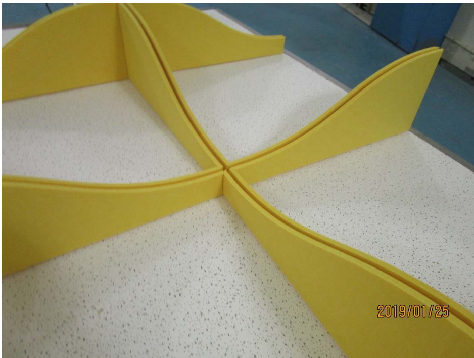
Figure 2 – Detail of fissured ceiling tile, typical Switchblade joint
