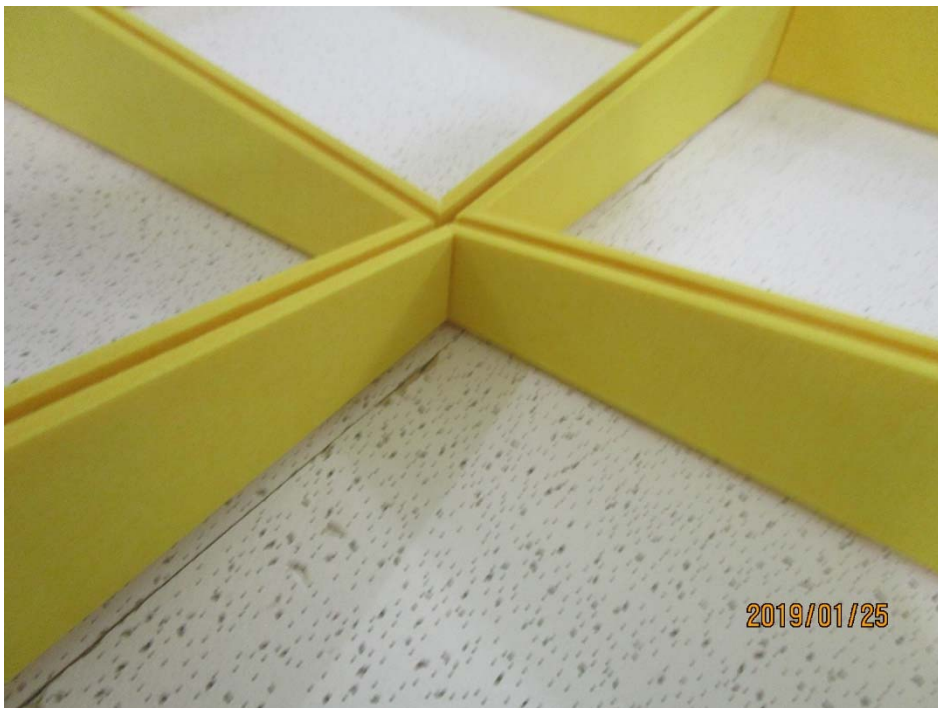
Figure 2 – Detail of Layer 1, typical Switchblade joint
