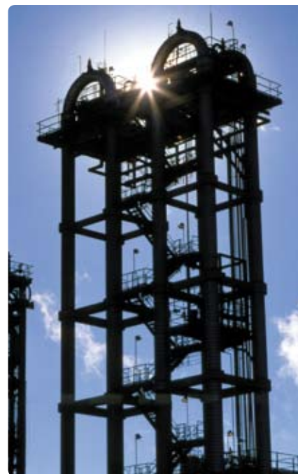
Figure 13: The characteristic Spheripol double loop.
