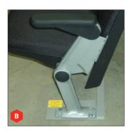
B. When removing the gang of chairs, install bolts into the threaded anchor inserts in the floor, so debris will not fill the holes. See Assembly Instructions for hardware use, and replace any missing or damaged hardware.
