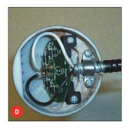
D. With the housing hanging on the conduit, pull the two pins from the sockets in the element, remove the two screws holding the element in place and remove it. Finally, remove the flexed mylar window from the slots in the old element and reinstall the window similarly in the new element. To reinstall the aisle light, reverse the preceding steps. Turn on power supply and verify all aisle lights are properly working and safe.
