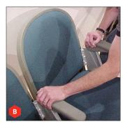
B. Try to move stanchion from side to side and front to back. Tighten anchors to the correct torque as specified in the Assembly Instructions. Replace any missing or broken anchors.
