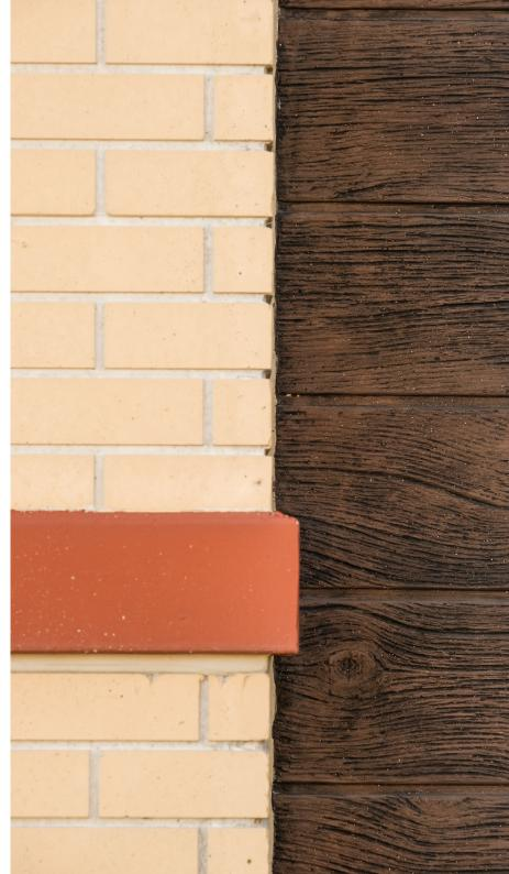
ABOVE: Nawkaw Stain Technicians transformed this road pump station near Christchurch, New Zealand. Stain was applied with a leatherlike finish on formlined concrete to create the final look.
