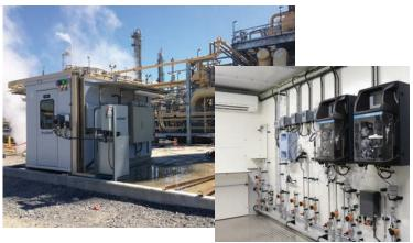
Weather and corrosion resistant cabinets for analysers and sensors.
