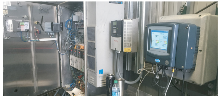
Hach Real-time Control for Sludge Thickening (RTC-ST) installed to help monitor and adjust chemical treatment, pH level and flow in a dairy facility's wastewater treatment plant.
