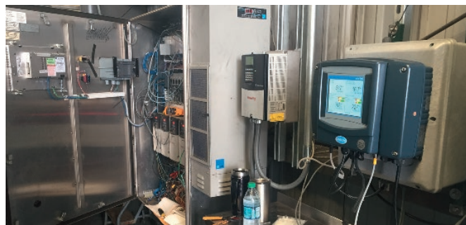
Figure 1: Hach Real-time Control for Sludge Thickening (RTC-ST) installed to help monitor and adjust chemical treatment, pH level and flow in a dairy facility's wastewater treatment plant.
