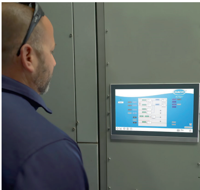
Examples of a typical RTC installation and RTC-DAF user interface screens. All settings, validity and fallback strategies are configured through the touchscreen and can be password protected.
