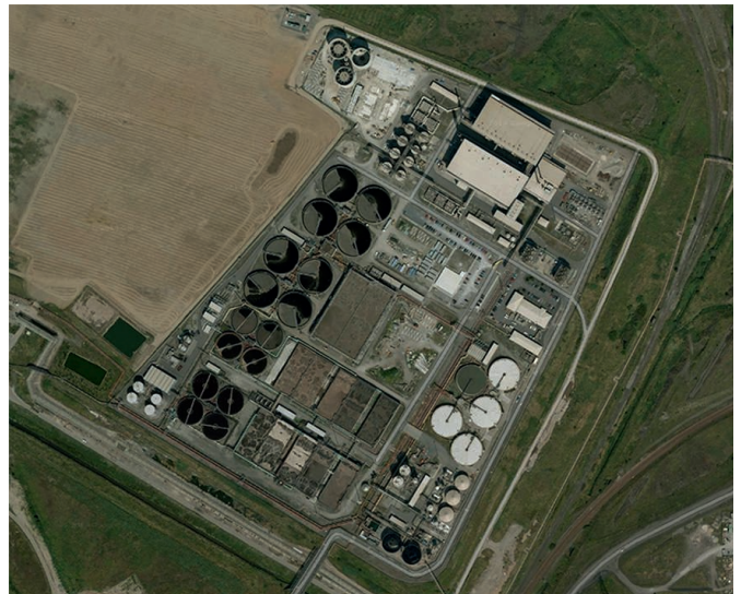
1. ábra: Bran Sands Wastewater Treatment
