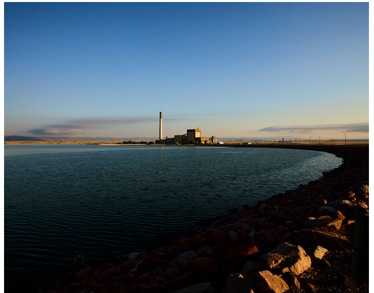
Fig 1: Platte River Power Authority's Rawhide Energy Station
