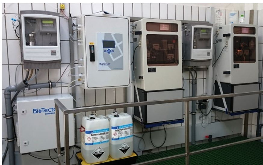
Figure 2: View of the measuring room with Hach® analyzers for TOC, phosphate, and ammonia, including sample preparation
