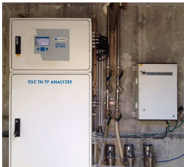
Figure 1: Installation of the Biotector B7000 in the analyzer house
