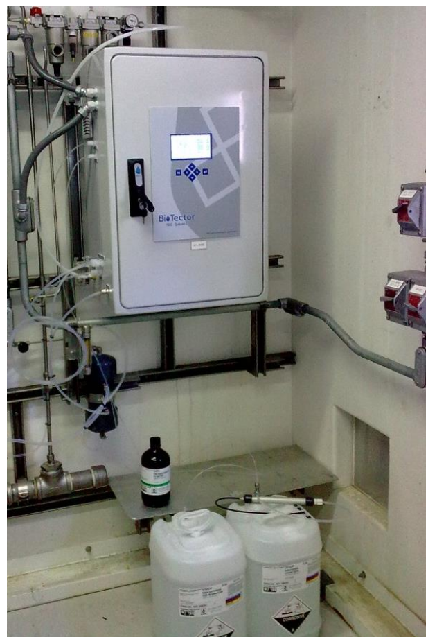
A typical installation of Hach's BioTector B3500dw TOC analyzers including a six-month supply of reagents and an instrument filter pack.
