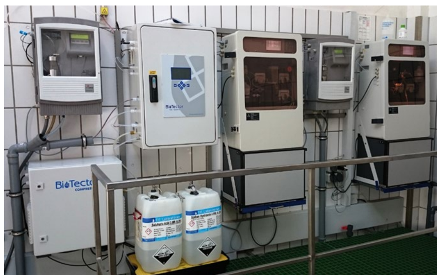
Fig. 2: View of the measuring room with Hach® analysers for TOC, phosphate, and ammonia, including sample preparation
