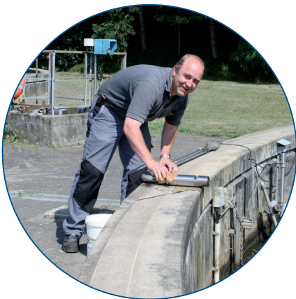
Fig. 2: Plant manager Gerold Thiemann has everything under control – including the NITRATAX plus sc nitrate probe.
