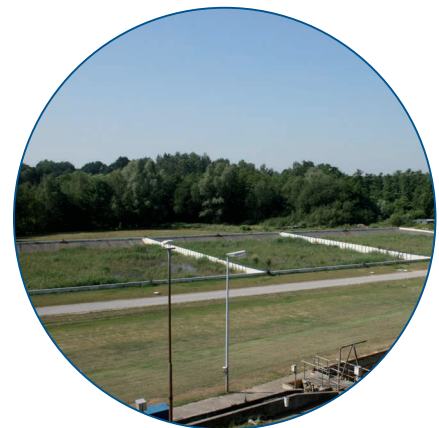
Fig. 5: View of the first sewage sludge soil humification facility in NRW
