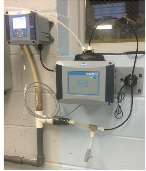
Figure 3: TU5300 sc process turbidimeter with flow sensor (optional) and sc200 controller installed at Western Berks DWTP
