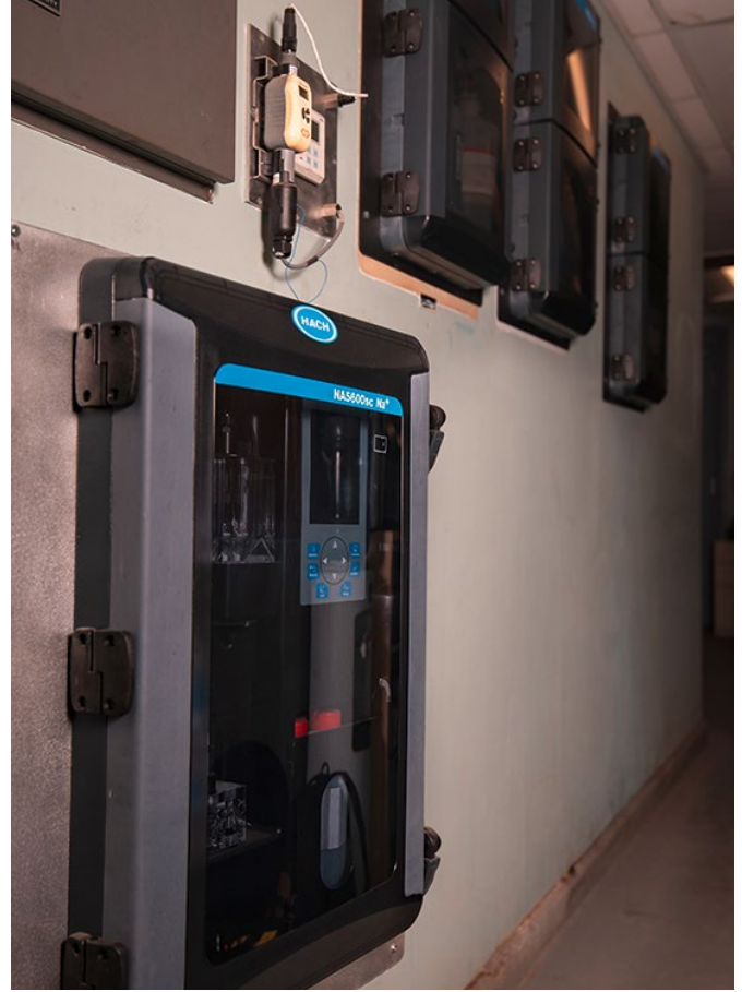
Fig 2: The Hach NA5600sc Sodium Analyser
