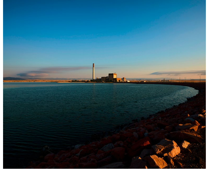
Şekil 1: Platte River Power Authority - Rawhide Energy Station tesisi
