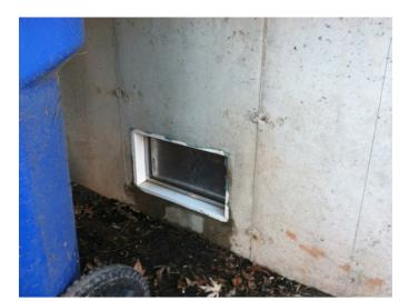
FAILED OPENING = INAPPROPRIATE ANCHORAGE
