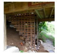
Round or square structures made of concrete or wood embedded in the ground.
