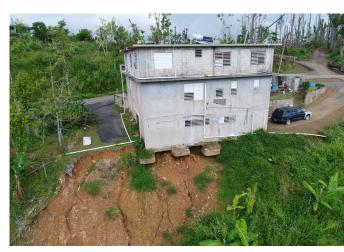
Failed foundation due to inappropriate soil
