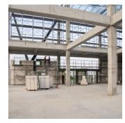
Columns, also called piers, are made of reinforced concrete and rest on footings.
