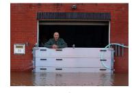
8. Permanently replace first floor doors with flood doors and install removable flood gates over entryways.
