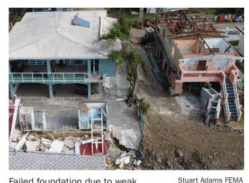
Failed foundation due to weak structural connections
