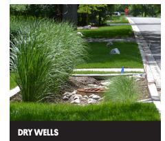
Dry wells are underground tanks, usually made of concrete, that store water to percolate or drain slowly to another site or sewer. Their design is similar to a pool.
