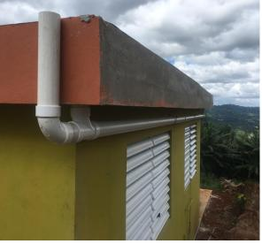
Materials used as catchment surface area and gutter should be free of pollutants like airborne chemicals that can leach into water.
