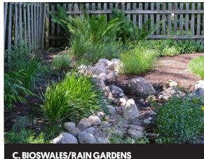
Bioswales/Rain Gardens receive water and filter it through different substrate layers and vegetation and help to absorb rainwater. They can be engineered to manage a specific amount of rainfall.
