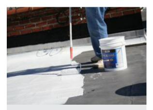
■ White or light colored roof surfaces that are highly reflective are recommended because they reflect heat from sunlight and prevent heat from entering a home and heating it up, while dark roofs absorbs sunlight which can heat up the home and surrounding site. Look for roof products or coatings with an aged solar reflectance greater than or equal to 0.55 which means that 55% of the heat is reflected away from the home keeping it cooler.
