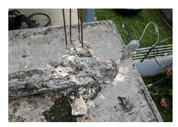
Failed foundation due to inappropriate concrete mix
