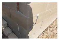
2. Seal all cracks and openings (except for flood vents or openings) below the DFE.
