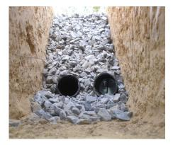
Install french drains around draining docks to collect and drain out excess water that reaches the foundation through the soil. French drains are perforated PVC pipes that are buried over a fine mesh and covered with gravel. For more info on French Drains, please refer to Strategy 1: Reinforce Site.
