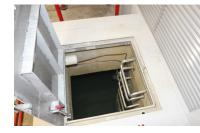
9. Install waterproof hatch doors on sidewalk hatches.
