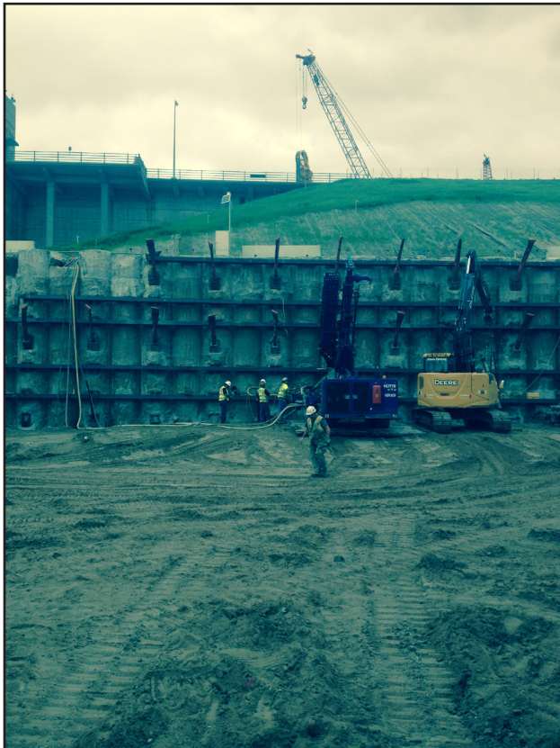
Figure 1: Tie backs on dam wall
