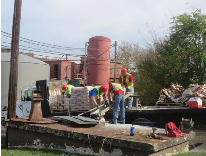
Well-site abandonment operations using 50-lb bags of HOLEPLUG® Graded Sodium Bentonite
