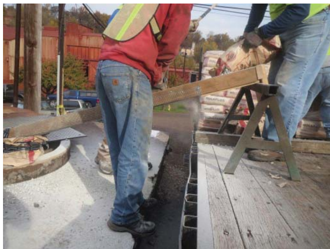
Technique of separating "fines" from \frac{3}{4} " HOLEPLUG® using screen trough. Note variable size of fine material below screen
