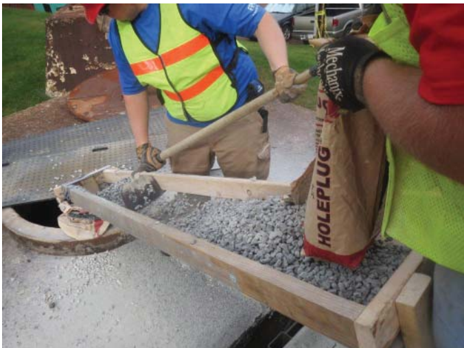
Pouring application of 3/4” HOLEPLUG® for well abandonment operations.
