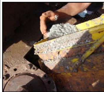
Addition of QUIK-GEL® GOLD bentonite and N-SEAL™ LCM
