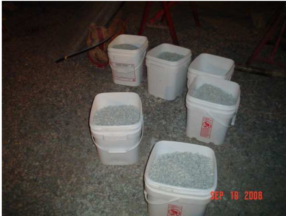
Screened Hole Plug 3/8" awaiting insertion to the hole.
