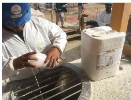
Figure 5. – Building lubrication fluid (left) – Addition of FUSE-IT in low concentration to reduce jacking force and skin friction (right)
