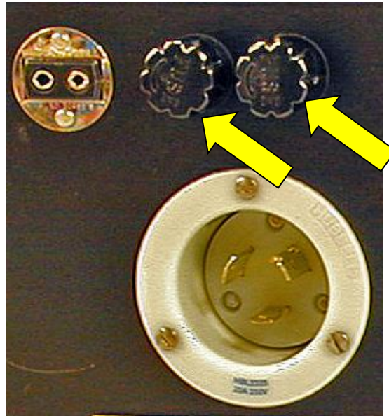
Figure 7-1 Power fuse holders
