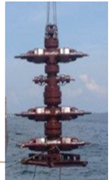
A modified surface capping stack is lowered onto the well to successfully cap and contain the well.
