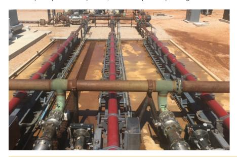
Each HPS unit meet unique requirements, including retrofit of existing pumps, and all programmed with automation controllers to efficiently move produced water to disposal.
